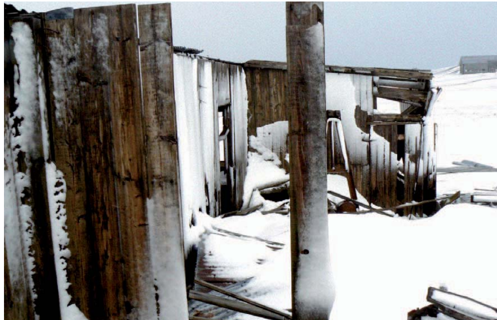
Figure 7. The north side of the dispensary at the end of a precipitation event showing accumulation of snow sticking to the wall boards. When this snow melts it is sufficient moisture to support fungal growth and decay.
