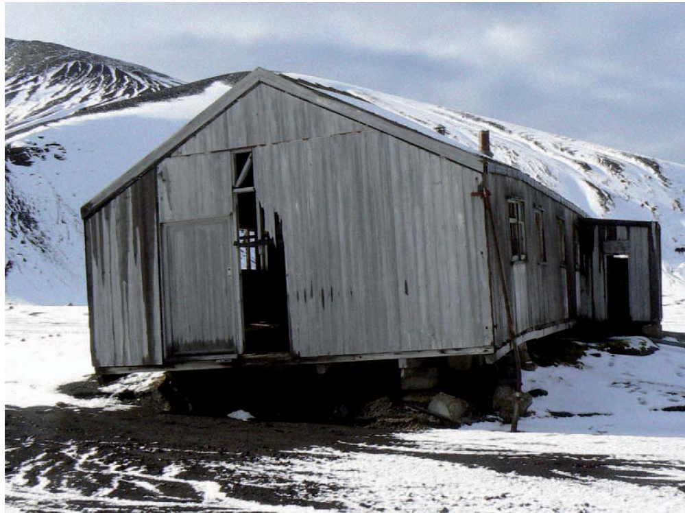
Figure 9. The Hunting Lodge has significantly less deterioration than other structures at the site partly due to a high foundation keeping the wood well above the soil. However the left corner shows erosion of the foundation that is in danger of collapse. Photo: Benjamin Held
