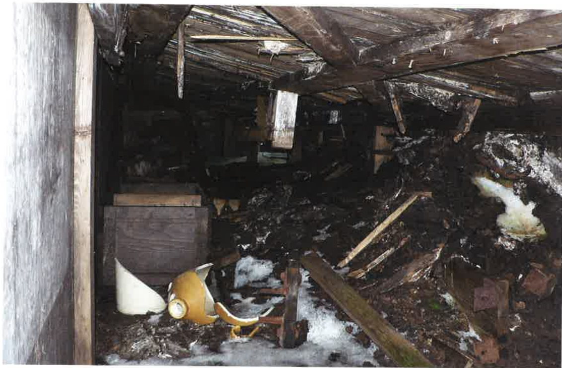
Fig. 2. The Main Building showing collapsing floor built by British Antarctic personnel from Base E. This floor was built 4 feet above the original floor and covers historic artifacts, debris and ice. Photo: Brett Arenz
