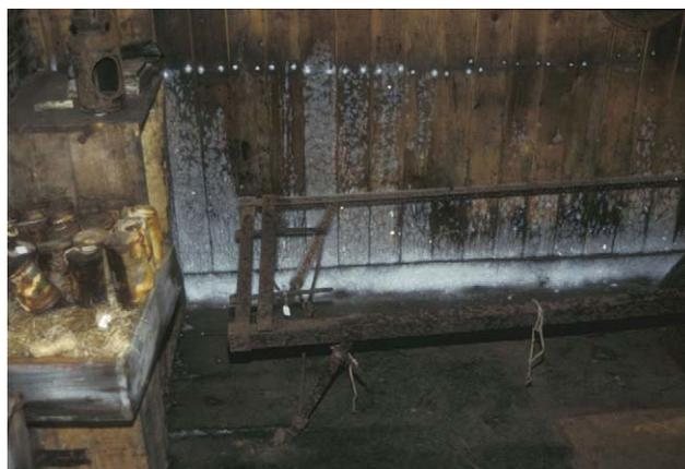
Fig. 4. Frost accumulation inside Cape Evans hut at the base of the south wall in the galley. When temperatures rise above 0°C the frost melts producing sufficient moisture for mold growth in this area.
