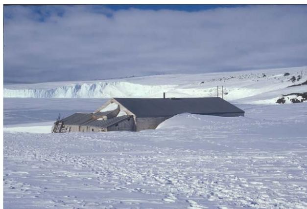
Fig. 5. Cape Evans hut in mid December showing a large amount of drifting snow that accumulates over the winter months.
