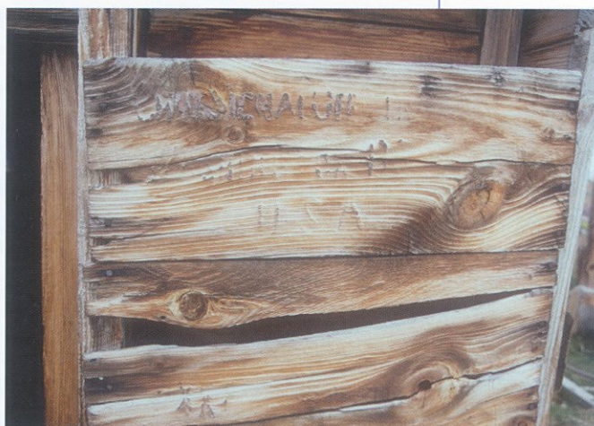
The effects of wind erosion on outer boards of Dedrick's hut cause deep grooves in the wood. The less dense earlywood cells of the wood are eroded faster than the latewood cells resulting in a grooved appearance. An inscription, "CHIEF SIGNAL OFFICER/WASHINGTON DC USA" placed on this reused wood during the Greely expedition (1881) has partially resisted the effects of the wind.
