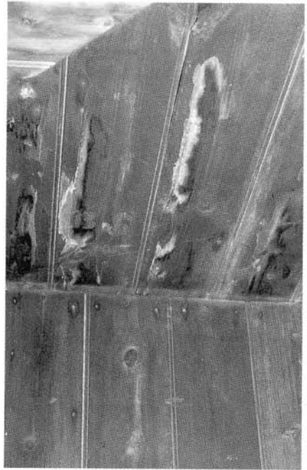
Fig. 4. Deterioration in Scott's Discovery hut at Hut Point. 4a (top left). View of hut and veranda. 4b (middle left). Snow accumulation under veranda and salt accumulation on lower exterior boards on side of hut without veranda facing the Ross Sea. 4c (bottom left). Salt accumulation and defibration of exterior boards near the ground on hut. 4d (top right). Salt accumulation on ceiling inside hut.
