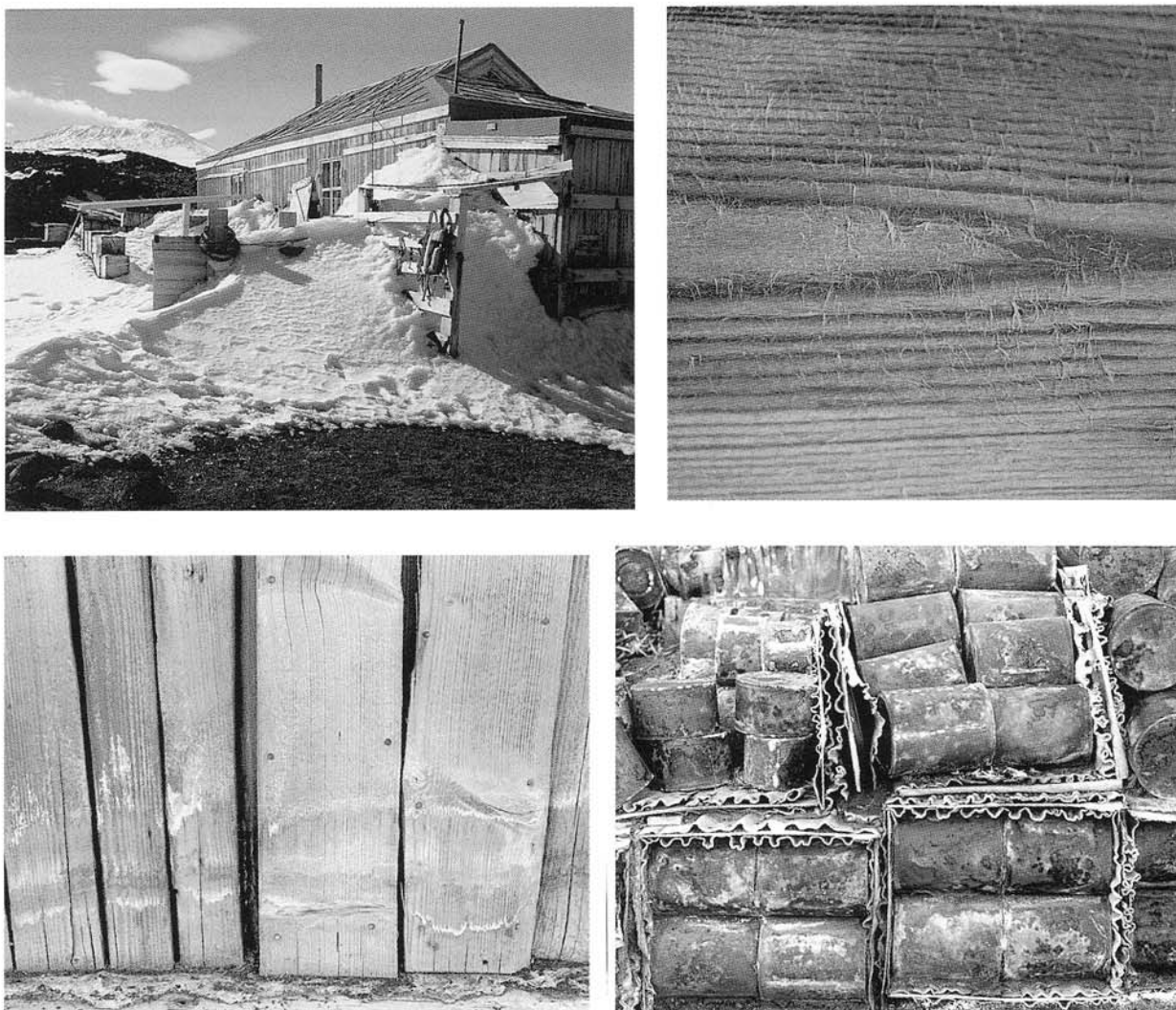
Fig. 3. Deterioration in Shackleton's hut at Cape Royds. 3a (top left). View of drifted snow covering the side of the hut. 3b (top right). Defibrated board from a wall inside the porch of the hut, showing loosened surface fibers on the wood. 3c (bottom left). Salt accumulation on exterior boards of hut near ground. 3d (bottom right). Delaminated and defibrated wood boxes outside of the hut. These plywood or 'Venesta' crates made out of birch wood have defibrated surfaces.
