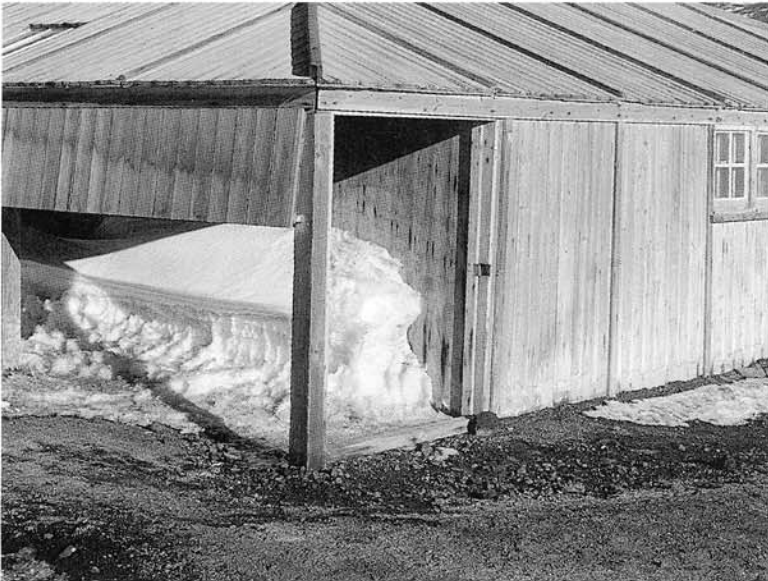
Fig. 4. Deterioration in Scott's Discovery hut at Hut Point. 4a (top left). View of hut and veranda. 4b (middle left). Snow accumulation under veranda and salt accumulation on lower exterior boards on side of hut without veranda facing the Ross Sea. 4c (bottom left). Salt accumulation and defibration of exterior boards near the ground on hut. 4d (top right). Salt accumulation on ceiling inside hut.
